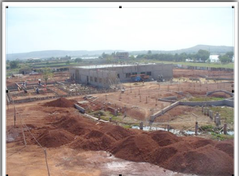
DEC 19, 2009 – View from the water tower overlooking the site
